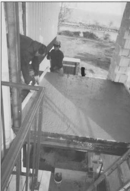
Smoothing out the cement floor. Photo by Ken Lay.
