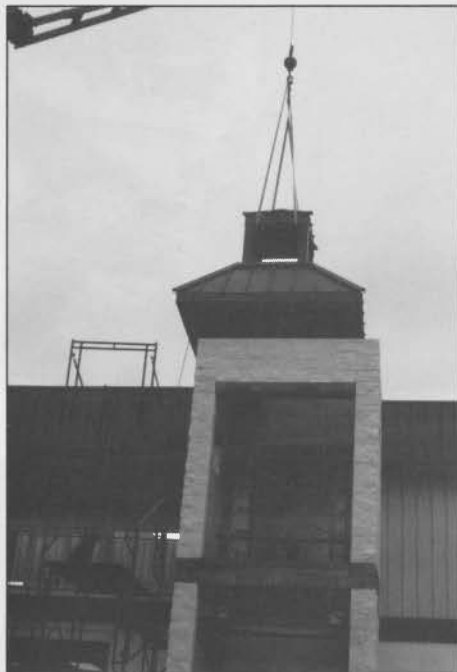
The roof is set in place with a crane. Photo by Ken Lay.
