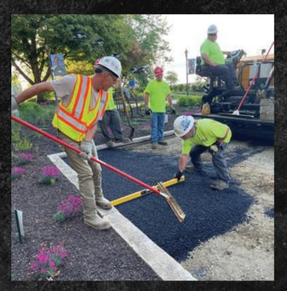
Mark Dolan, DXI Construction project foreman (orange bordered safety vest) ensures that the new pavement will have the fall to enable proper drainage
